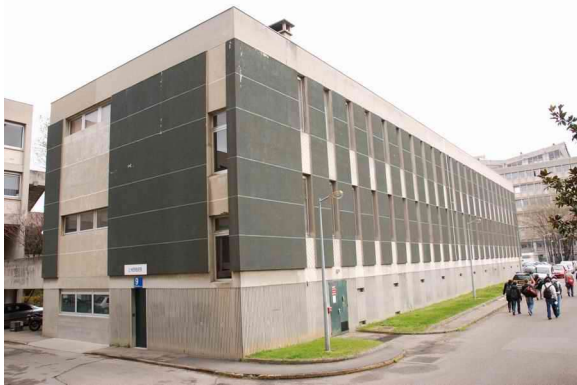
Salle Guilliermont – "l'Herbier" Building
